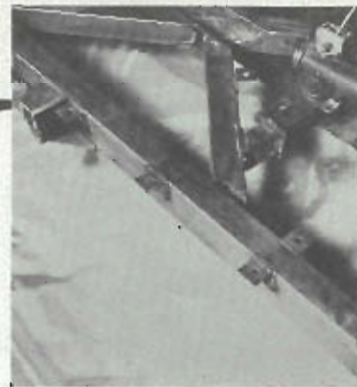
Body brackets installed
